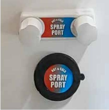
On the utility center panel is a hot cold mixing valve. Set the temp here and plug the sprayer in any one of three locations for the perfect temperature spray.
